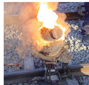
Welding railroad track with Thermite
