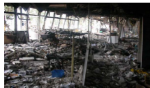
Figure 1: Selection of relevant photographs indicative of the damage on the building No 5 (front of the building – inside laboratory room – collapse of the floor).
