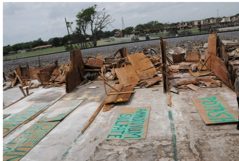
Facility and storage bins constructed of combustible materials
