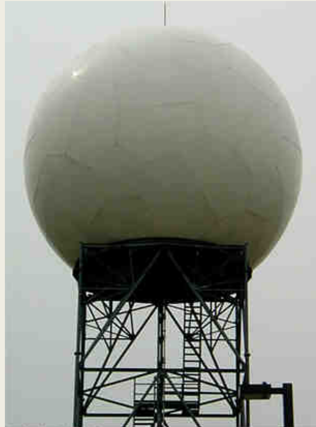
Typical NEXRAD Doppler radar tower
