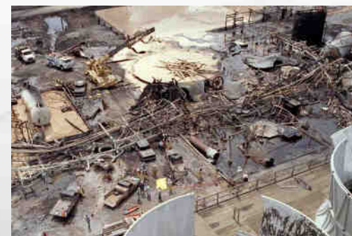
Arco Chemical (1990) 17 Dead; 5 Injured; $36 MM in damage
