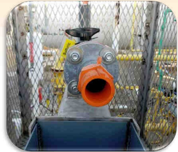
New coupling on the sulfuric acid fill line (Source: MGPI)
