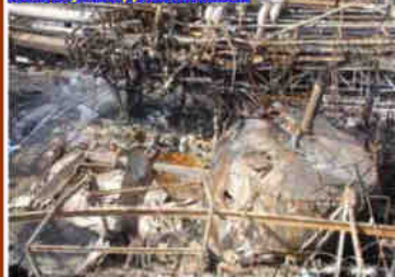
Photo 1: Destroyed AA Tank
